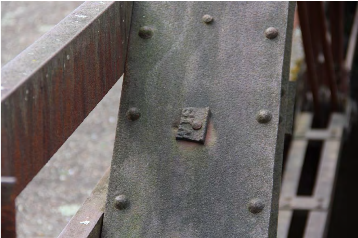
Photograph 10 of 11. Detail of bridge plate fragment.
