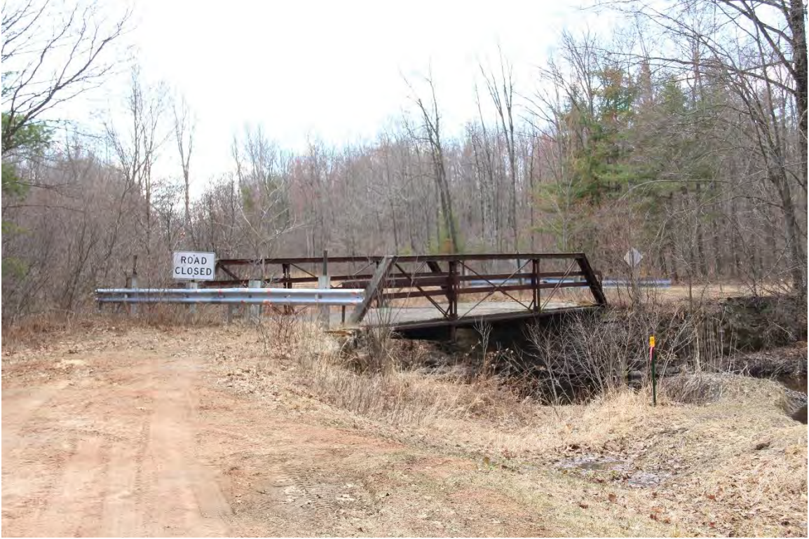
Photograph 1 of 11. Overview, approach, and northwest elevation, view facing south.
