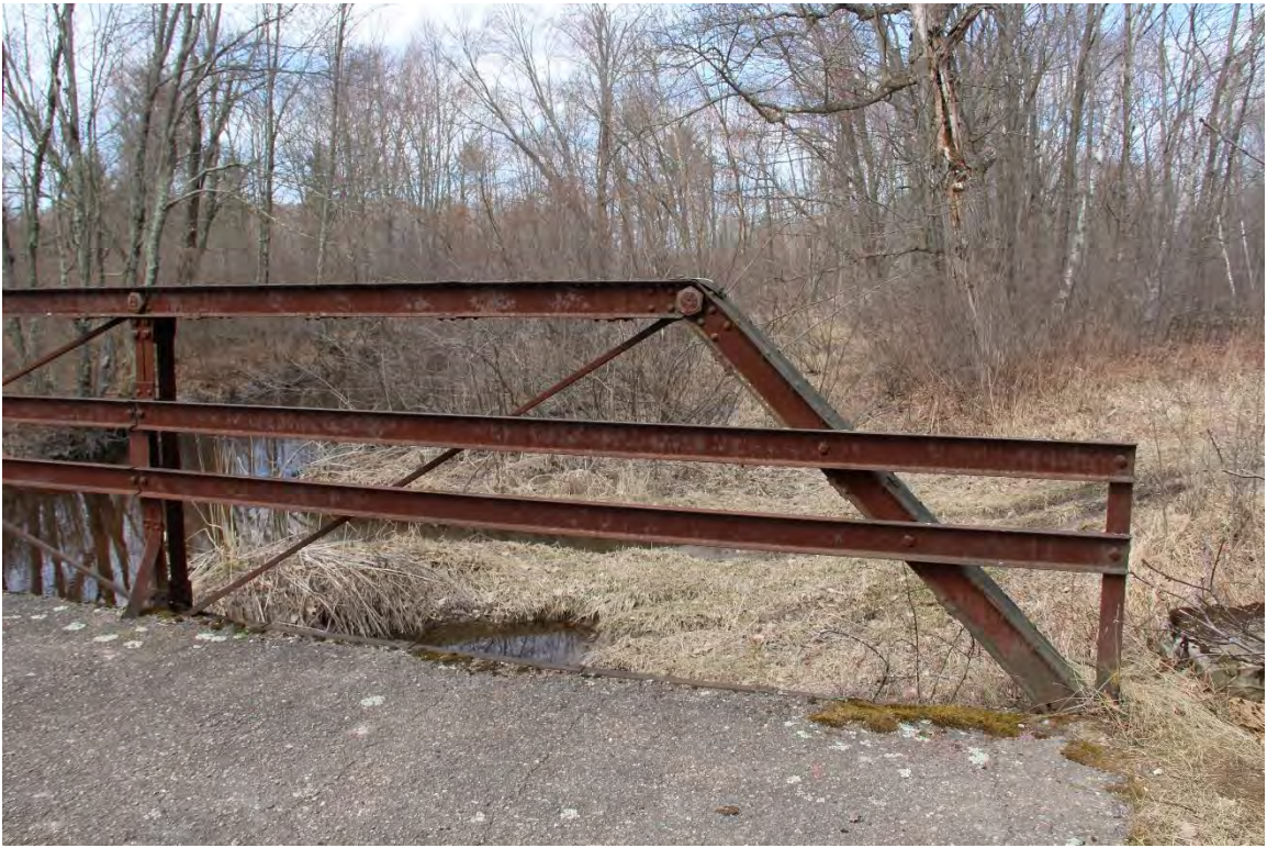
Photograph 9 of 11. Bridge railing, view facing northwest.
