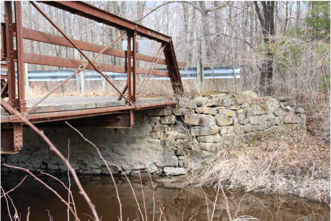
Photograph 8 of 11. Northeast stone abutment and wingwall, view facing north.
