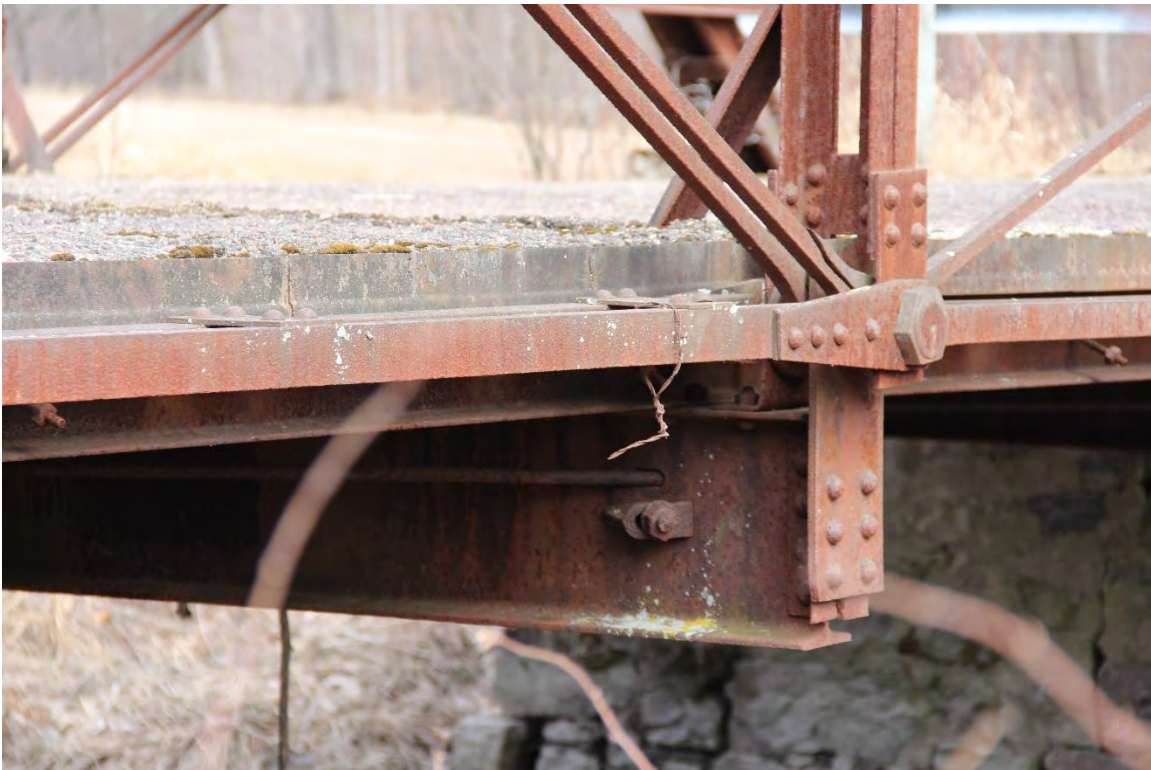
Photograph 6 of 11. Detail of pinned connection where bottom chord, main verticals, diagonals, and floorbeams meet.
