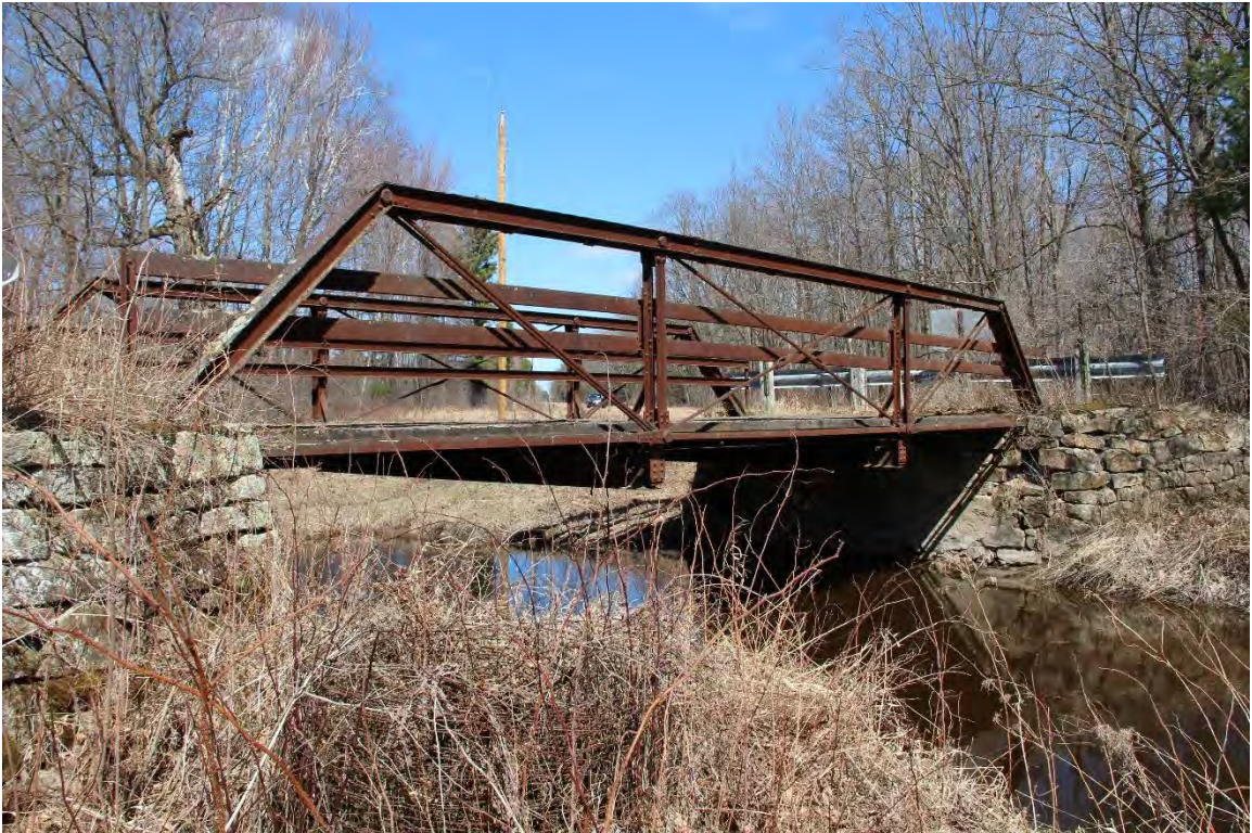
Photograph 2 of 11. Southeast elevation and abutments, view facing north.
