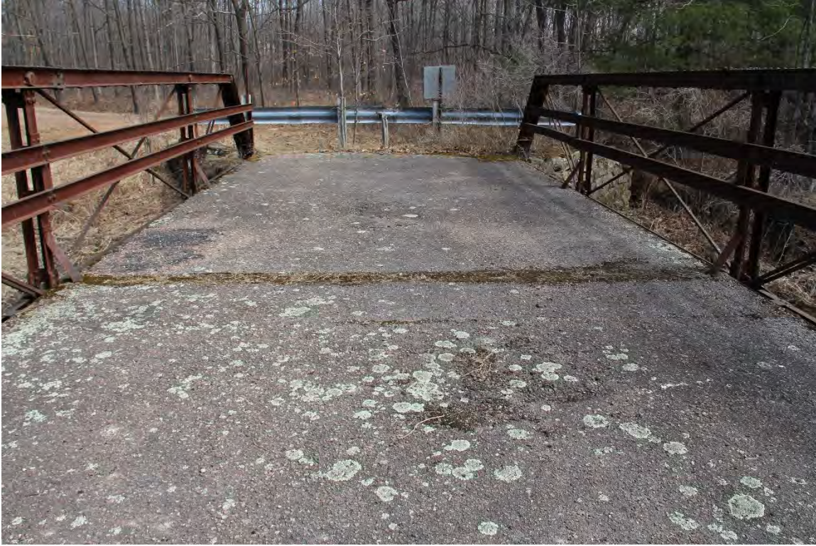
Photograph 11 of 11. Replacement deck with bituminous surfacing, view facing northeast.
